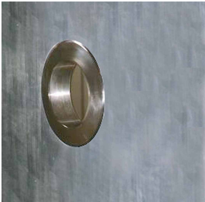
Figure 3: Adaptor seen from inside the tank
