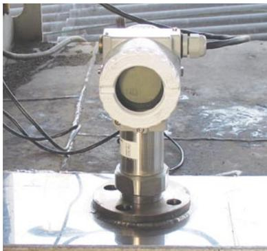
Smar guided wave Radar transmitter
