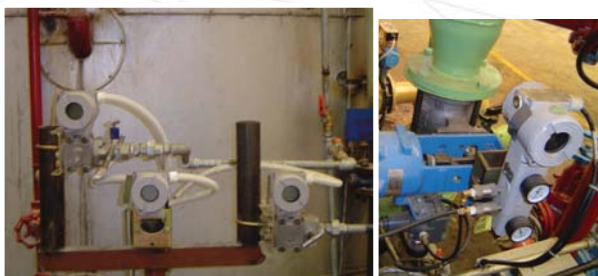
Details of Field Equipment Installation
