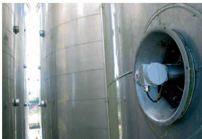
Figure 4: DT302S Installed on a Fermentation Tank
