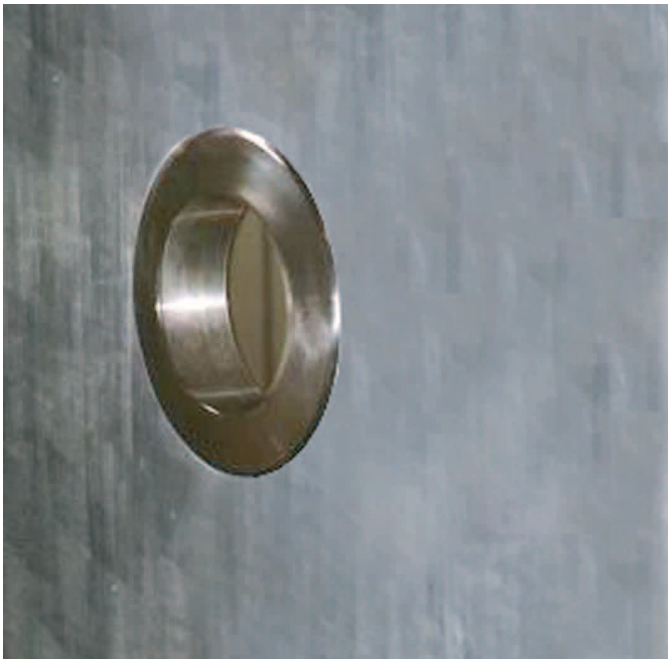
Figure 3: Adaptor seen from inside the tank
